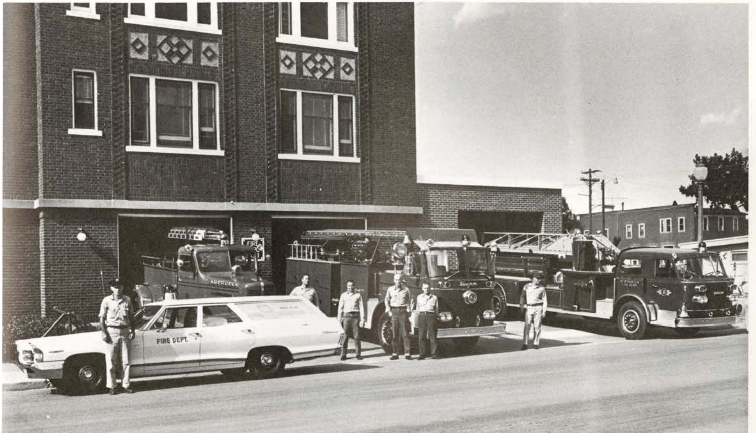
Two well-equipped fire stations offer good fire protection to Aberdeen residents and businesses
