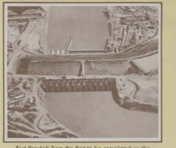
Fort Randall Dam, the first to be completed on the upper Missouri River, is impounding water and will be in full operation by the first of next year.
